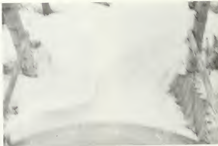
Looking down into WEST ENTRANCE Drifted in and unusable
